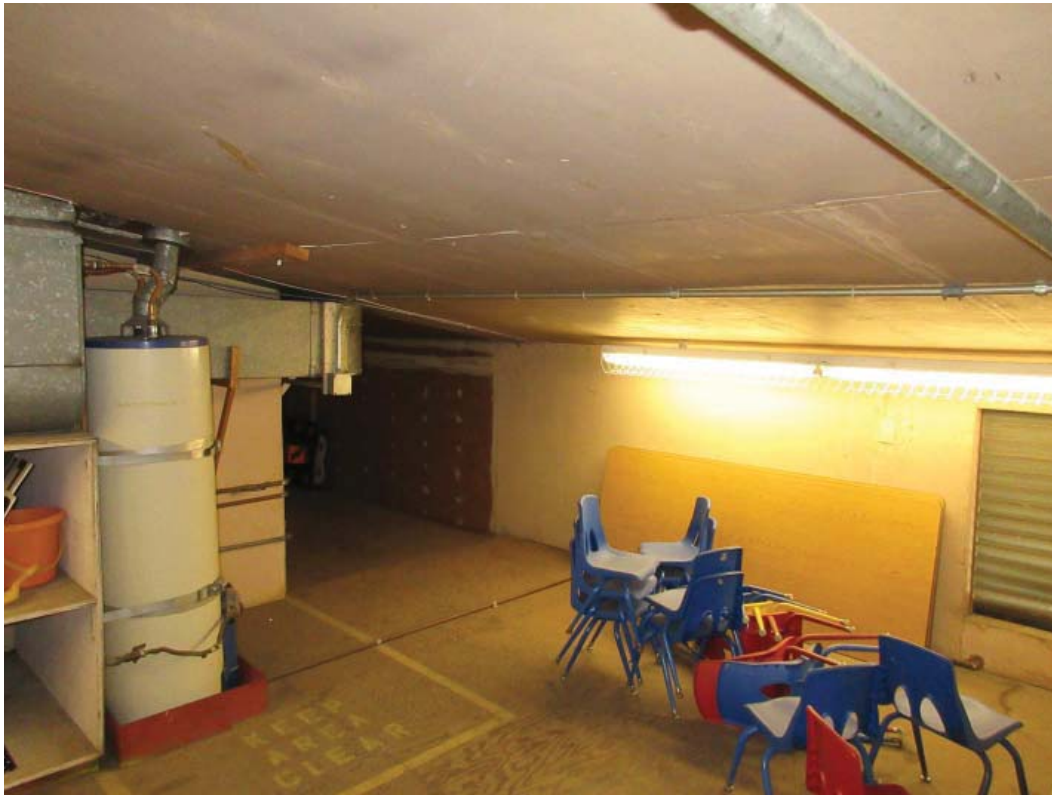
Photo 12 – South attic above the rest rooms.
