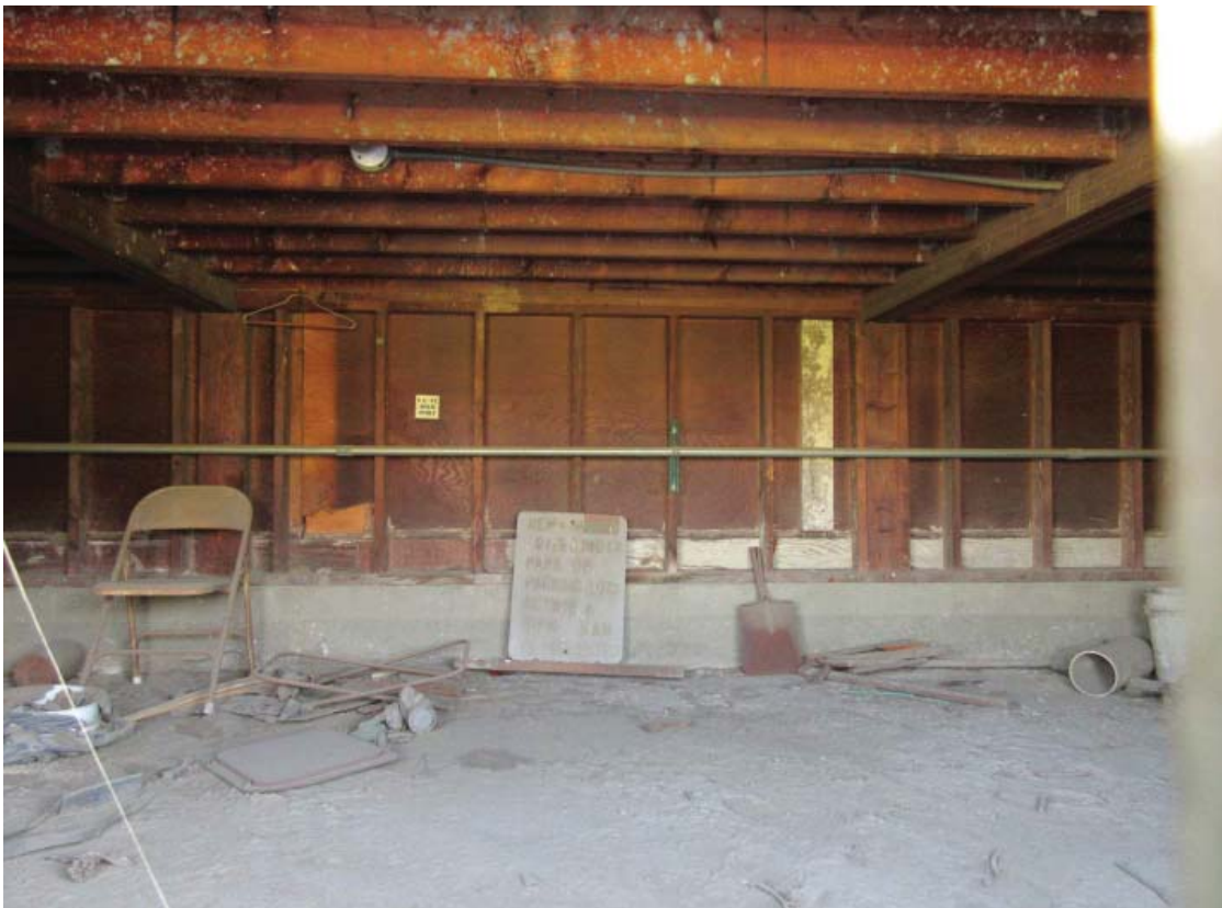
Photo 14 – East wall and wood framing below rear stage platform.
