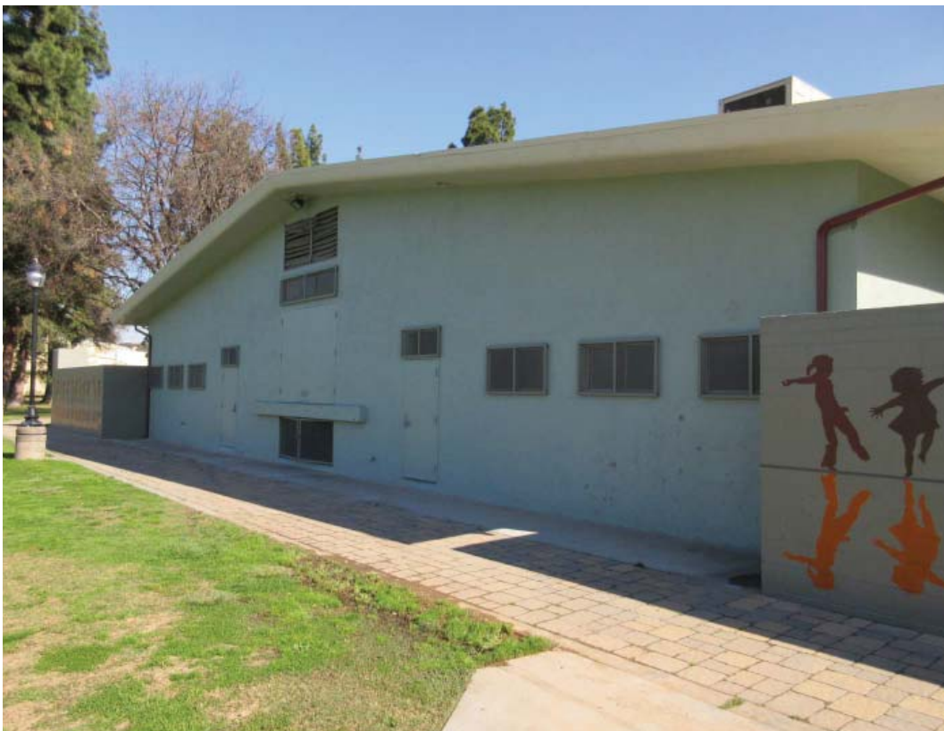
Photo 2 – Rear west elevation.
