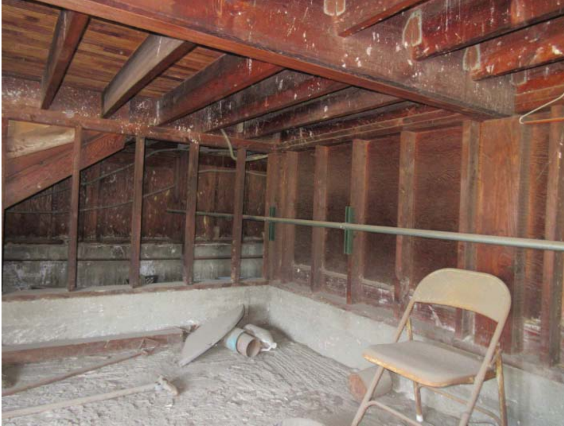
Photo 13 – North and east walls and wood framing below rear stage platform.
