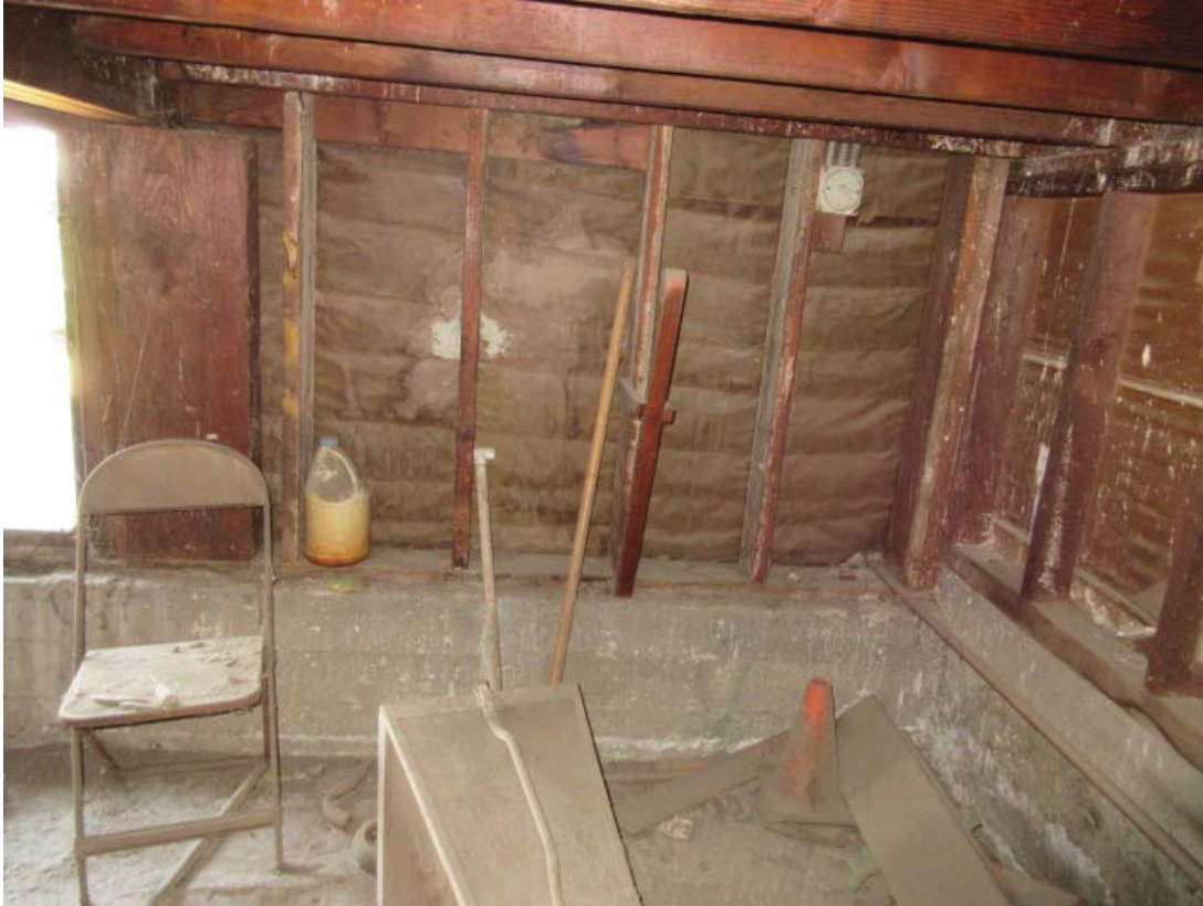
Photo 19 – West wall and wood framing below rear stage platform.
