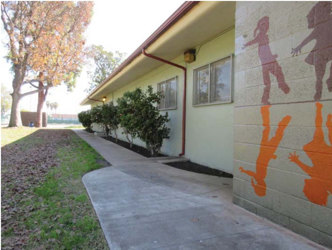
Photo 3 – Side north elevation.
