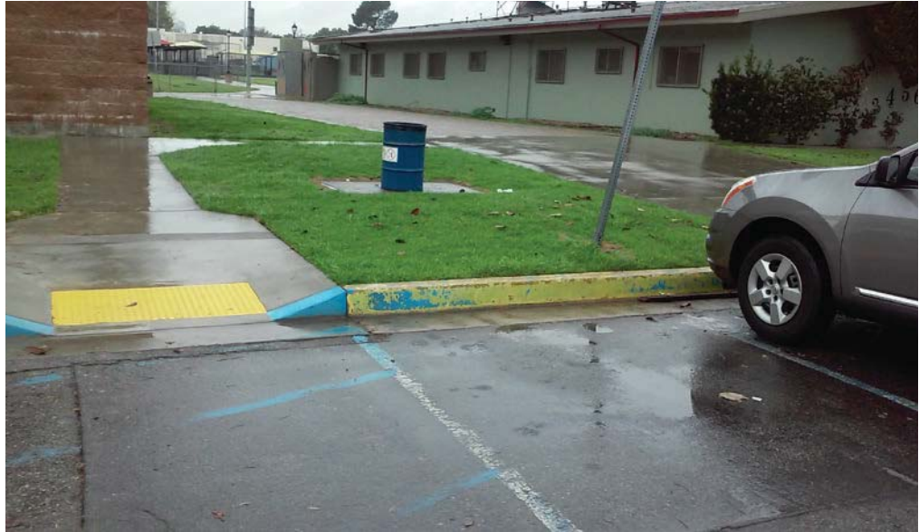
Figure 17: Picture of ADA accessible ramp.
