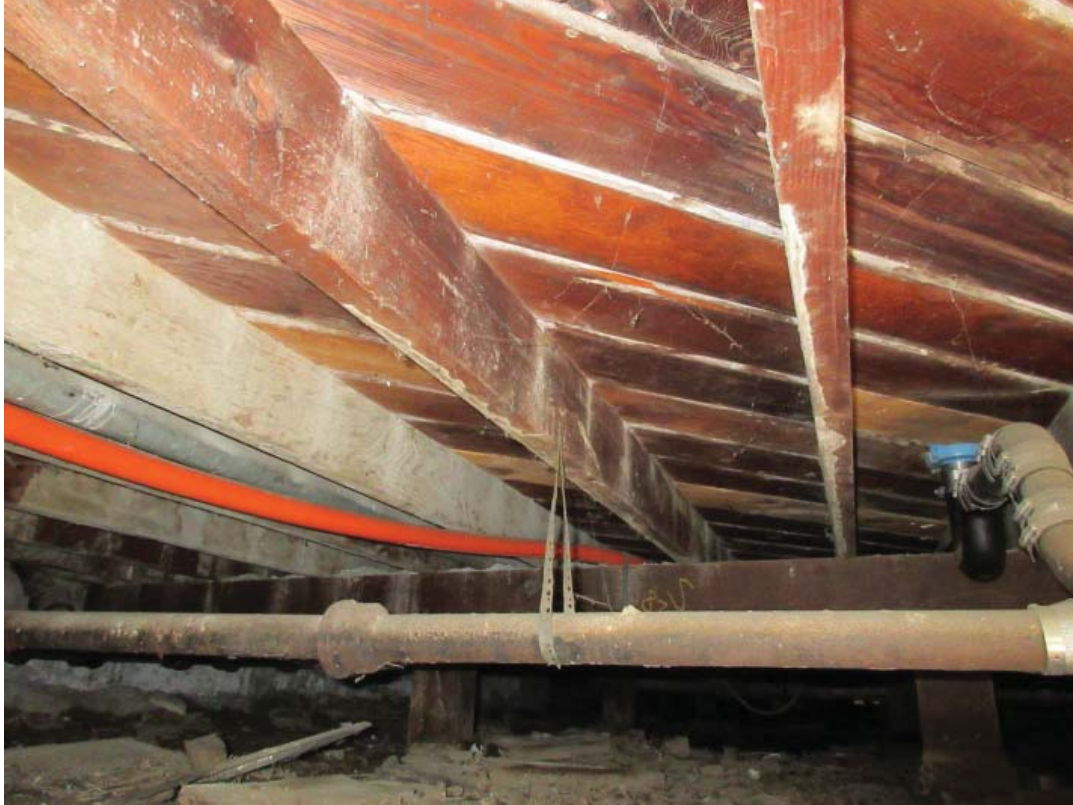
Photo 21 – Framing at south side crawl space below restroom.
