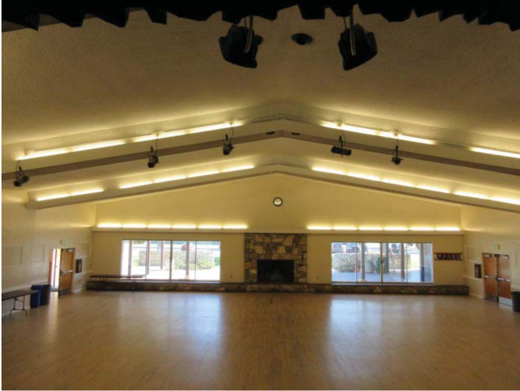
Photo 11 – Assembly room with steel bent frames above the ceiling.
