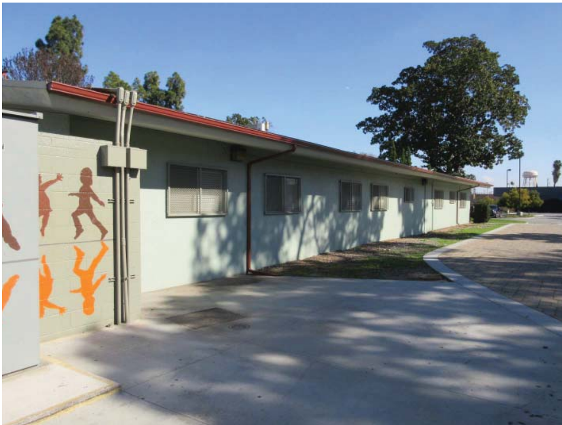
Photo 4 – Side south elevation.
