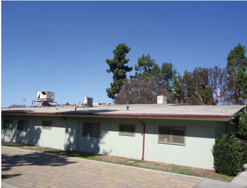
Photo 5 – Roof south elevation.
