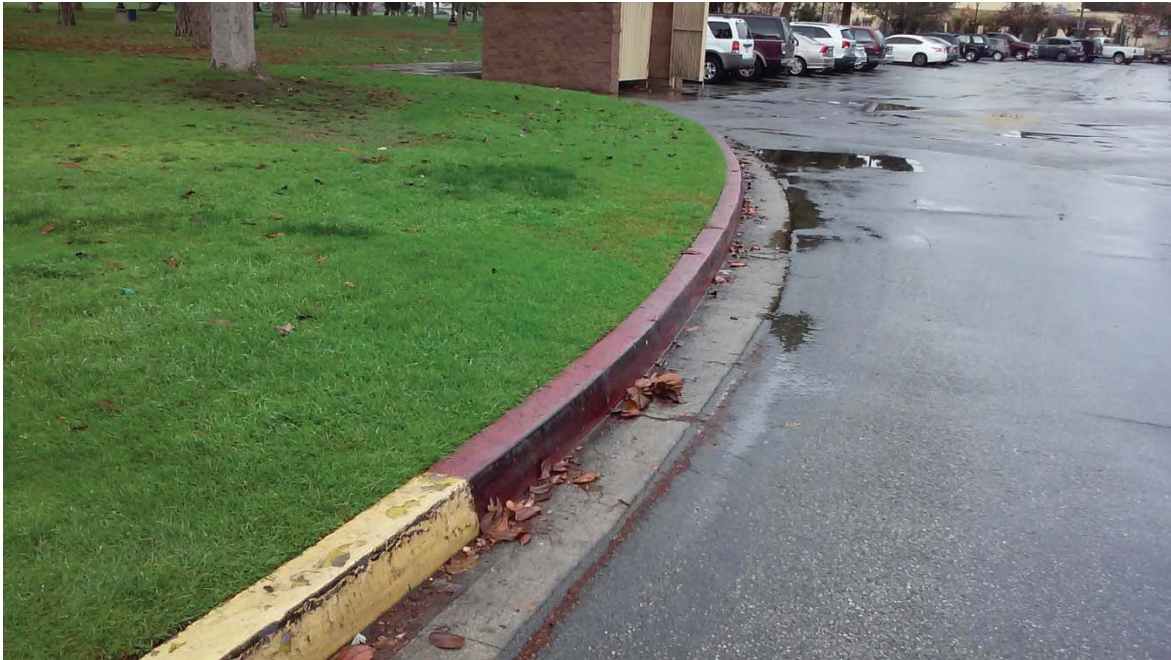
Figure 13: Existing Curb and Gutter on parking lot looking to the north.
