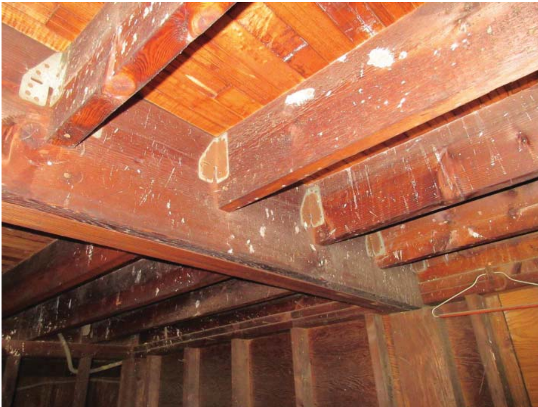
Photo 16 – Close up of wood framing below rear stage platform.
