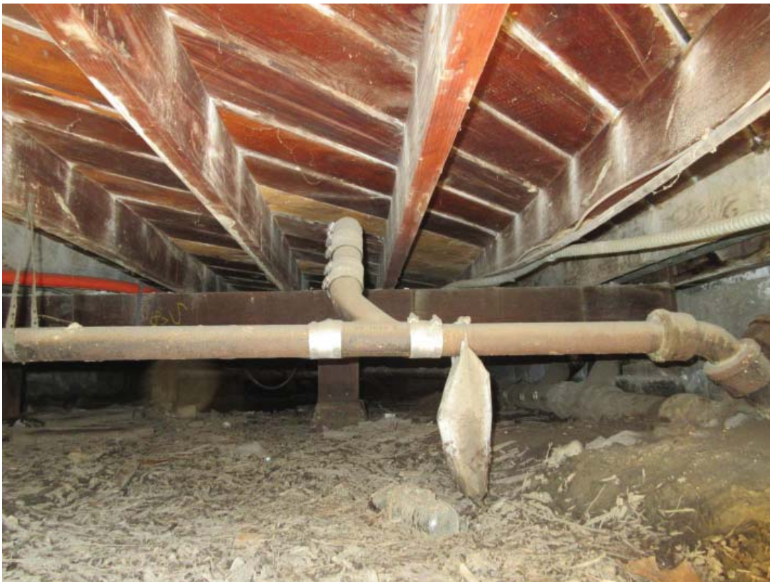
Photo 20 – Framing at south side crawl space below restroom.
