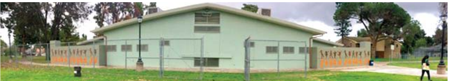
view of east wall
