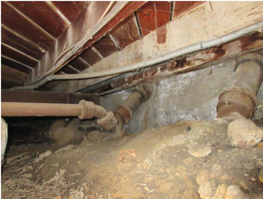
Photo 22 – Framing at south side crawl space below restrooms.
