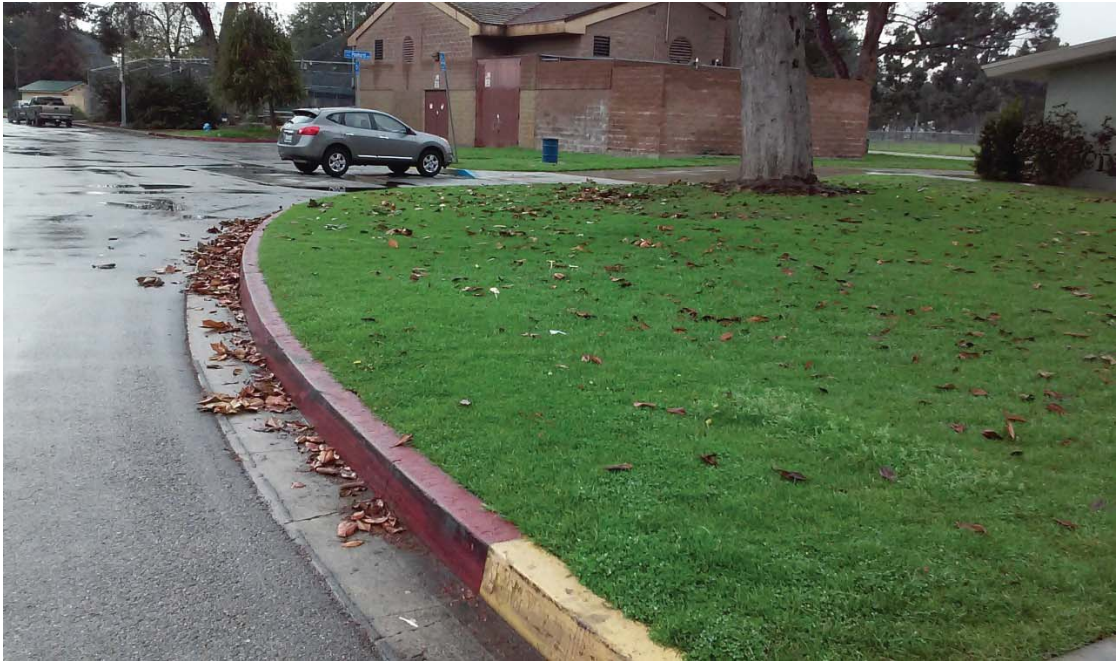
Figure 12: Existing Curb and Gutter on parking lot looking to the south.
